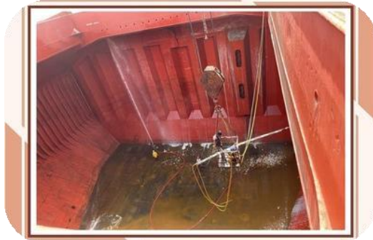
#3 Cargo Hold cleaning
